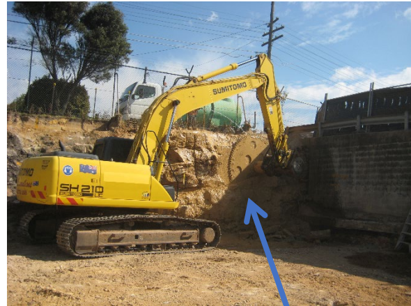
Rock Saw attachment was utilised to cut the sandstone face back
